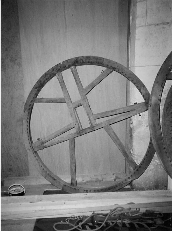
*One of the wooden 'ringing' wheels which provide the leverage for rotating the bells [M00107]*
