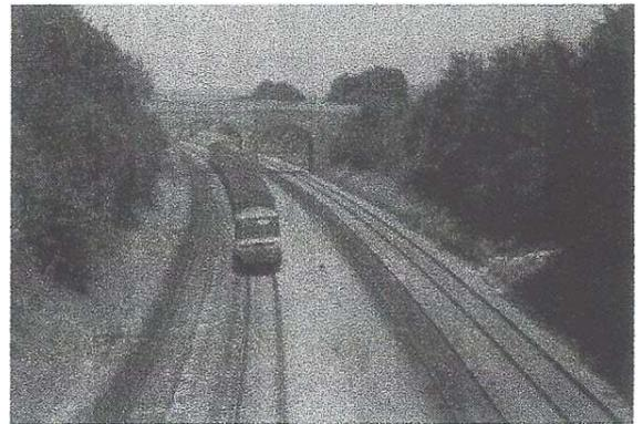
Purley Cutting - Note the two arches of the bridge over the railway at Purley Lane. The one on the left was built to span the broad gauge in 1837, while the one on the right was built in 1890 to span only a standard gauge line.
